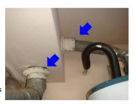
I recommend full evaluation of the flues connection, and replacing the collars with proper fire separation collars.
